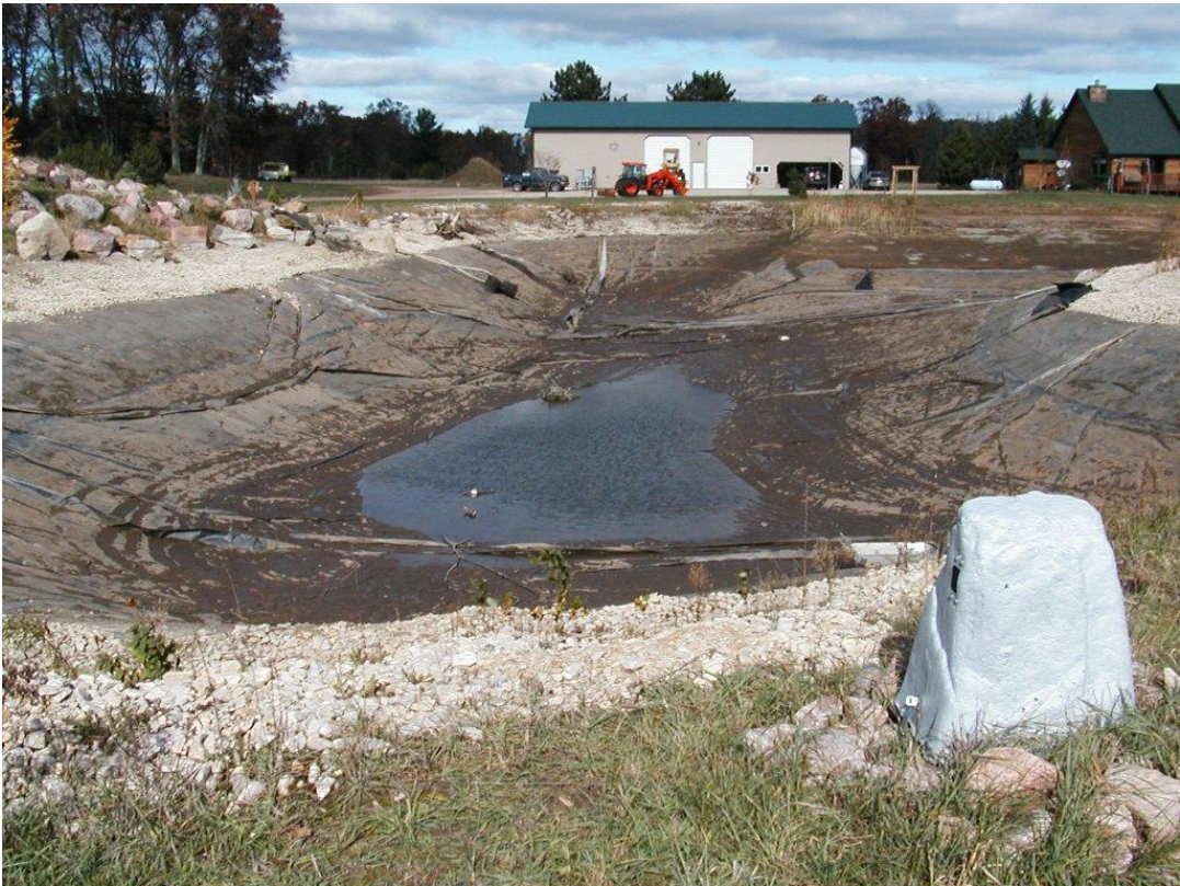
Figure 4: Deep half of the private pond following dewatering in fall 2007.
